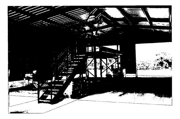
Interior View of Fuel Truck Loading and Unloading Shed showing Concrete Containment.
